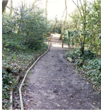
(2: The wooden leat collects excess water from the steep slope below Crescent Wood Road, to protect the path from erosion 3: The Ambrook stream flowing in its well-marked clay channel.)
